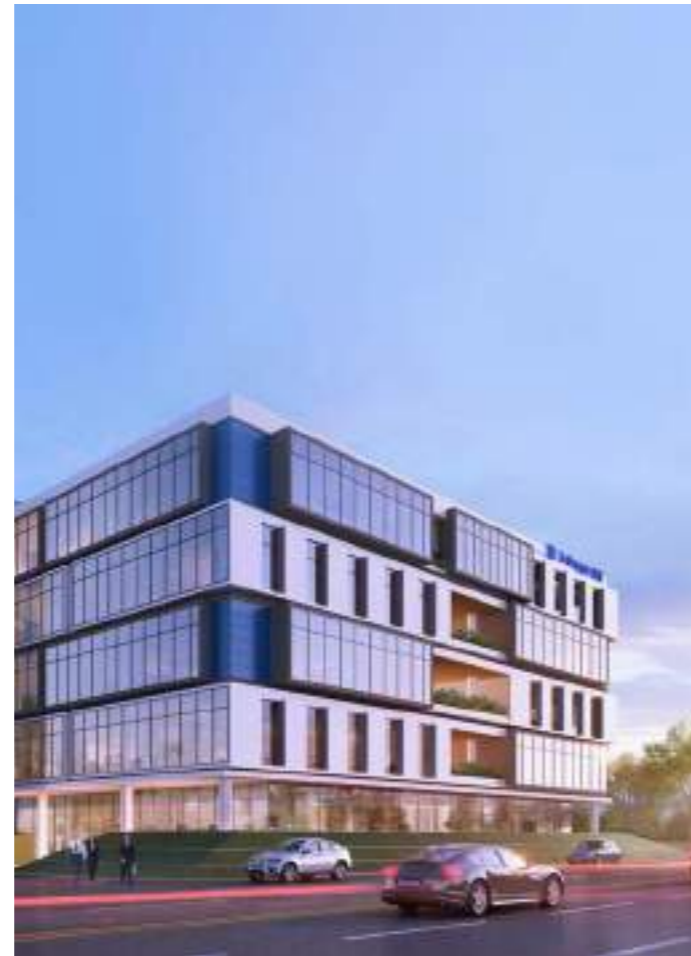
Unihopper R & D Building
