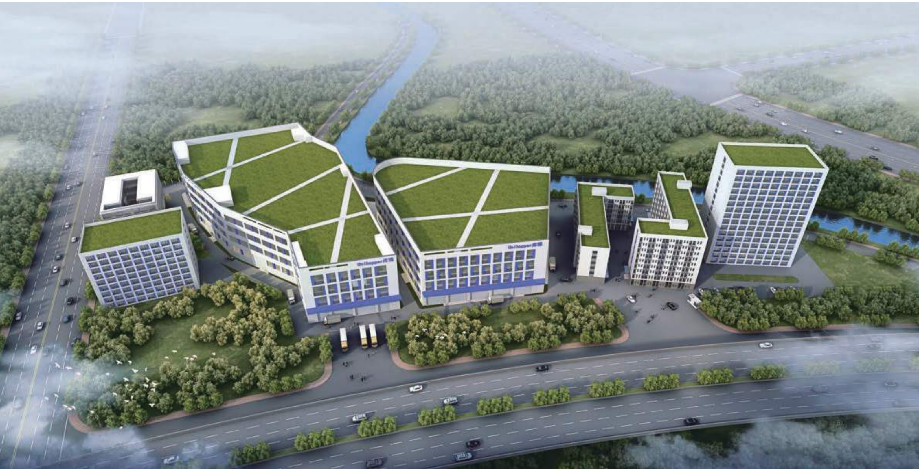
Unihopper Intelligent industrial park
