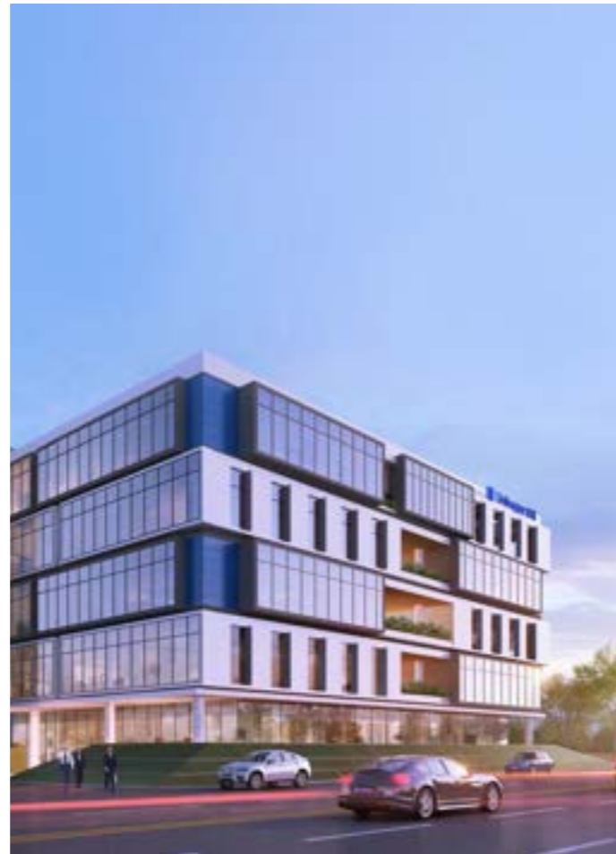
Unihopper R & D Building
